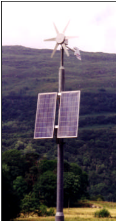
A low energy remote power site where a grid connection would otherwise cost thousands of pounds
